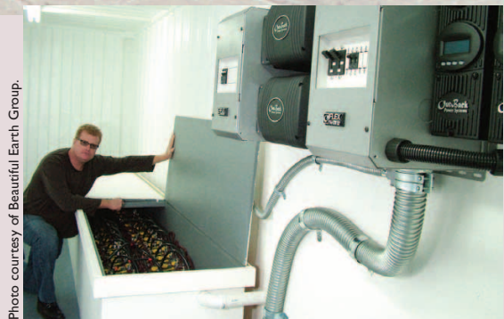
Beautiful Earth Group CEO Lex Heslin Shows Solar Charging Station's Trojan Battery System and Outback Inverters.
